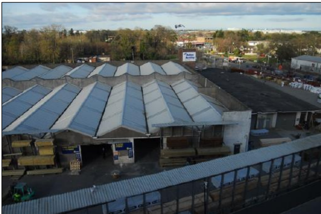
Oblique overview of the central part of the Study Area from the new development to the south, looking north
