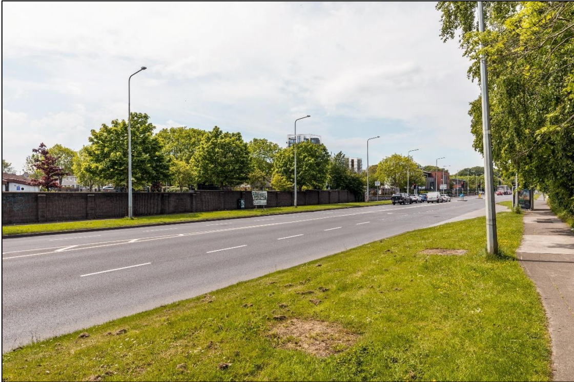
View 14.7: From Coolock Lane, looking west towards the subject site
