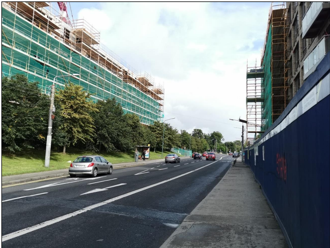
Figure 14.8: Photograph taken from Swords Road, south of site looking north towards subject site
