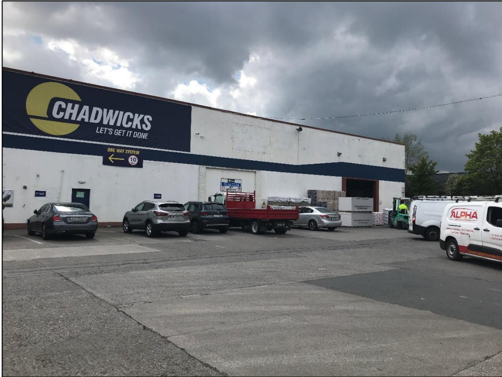
Figure 5.2: Buildings and artificial surfaces – BL3 habitat at the Site
